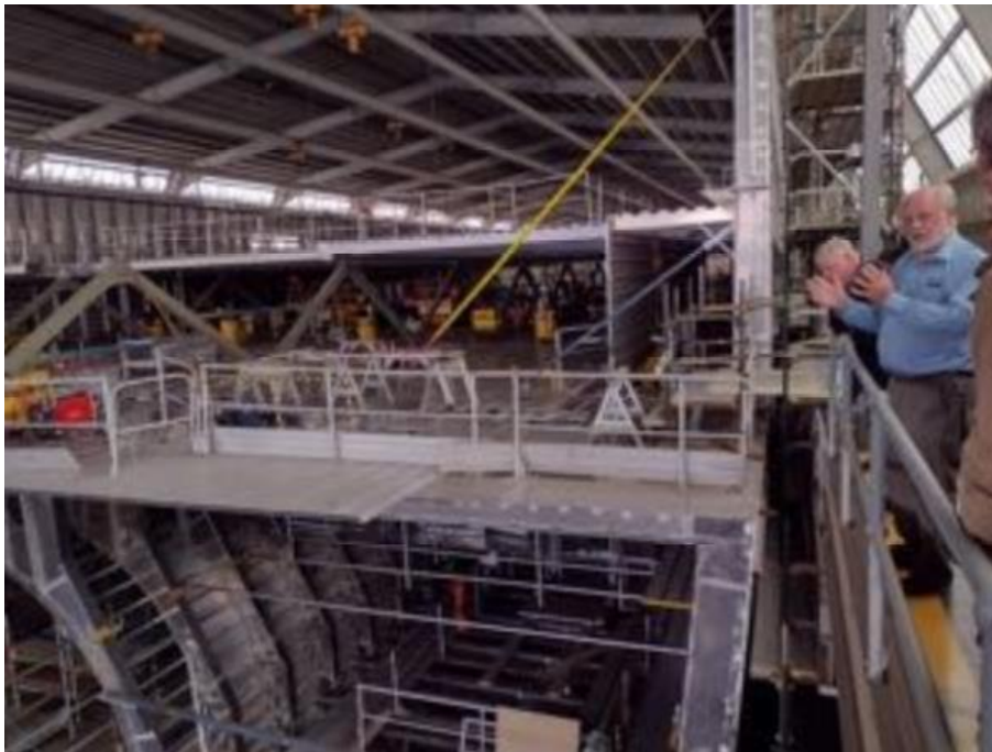
Robert Clifford and the ferry under construction
