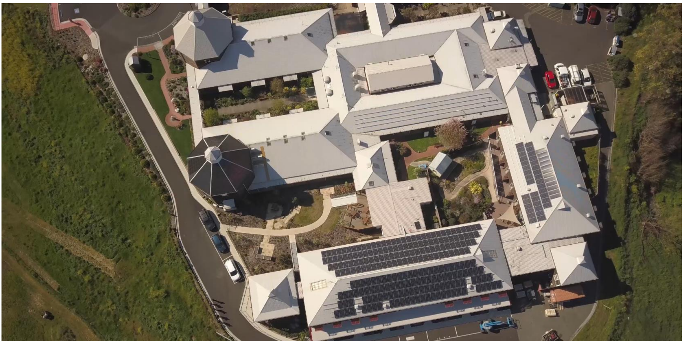
During the installation of 100 kW solar panel system at Corumbene
