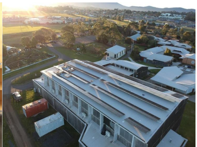
(L) The "Susteinerbles" volunteer student group (R) The new 100 kW solar panel system
